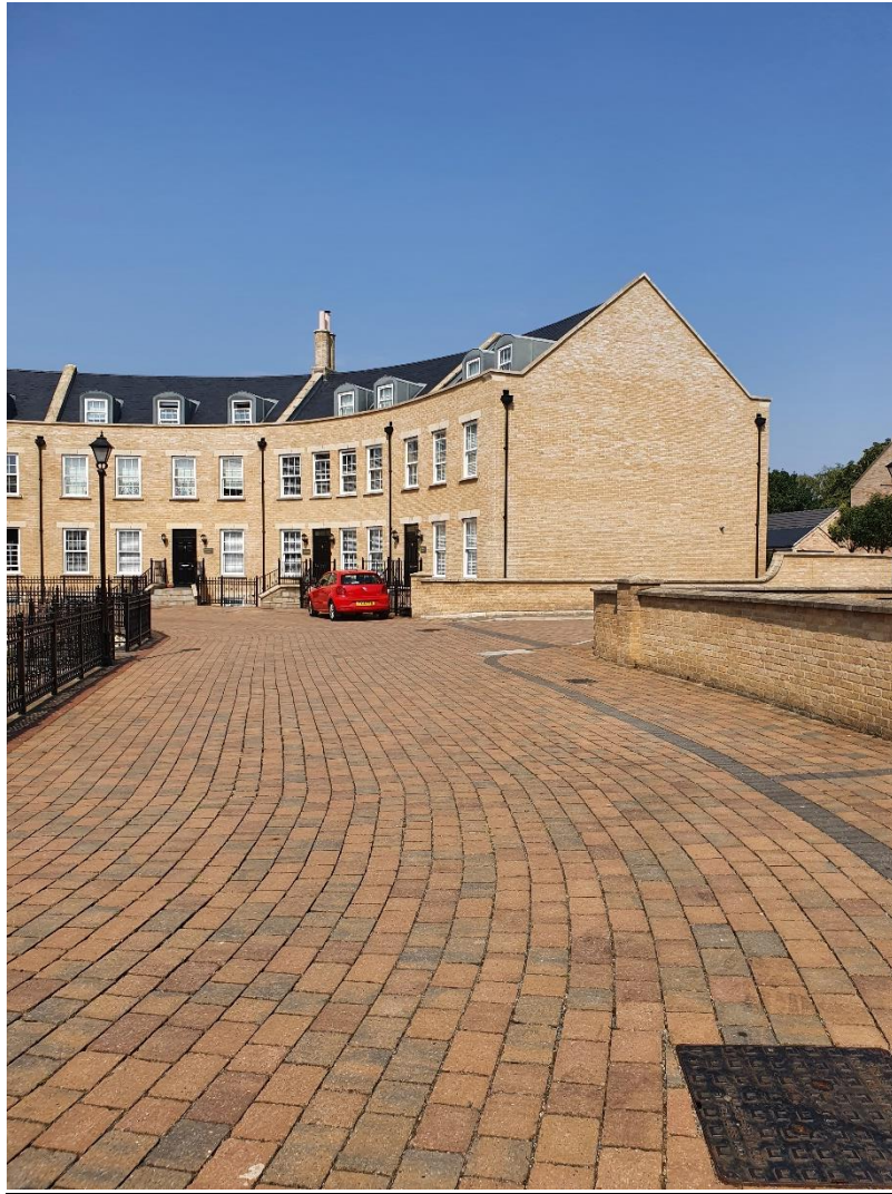
The application site and the opposite end of the crescent
