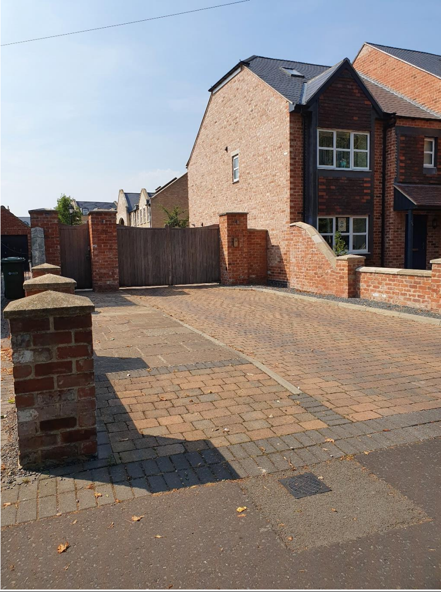
The access into the site
